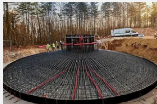
Figure 12 – An example of a gravity foundation
