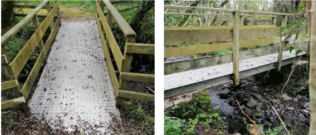
Figure 24: Mellons Glen Bridge
