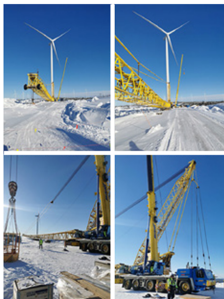
Figure 62: Main bearing exchange at Trattberget
