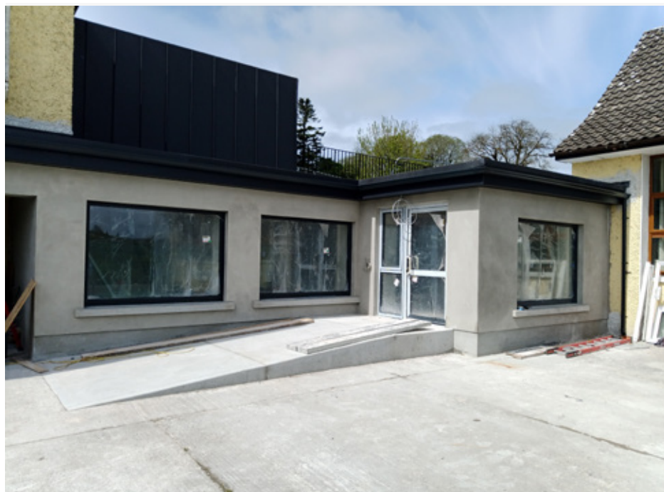
Figure 21: Scoil Mhuire Brosna link corridor in construction
